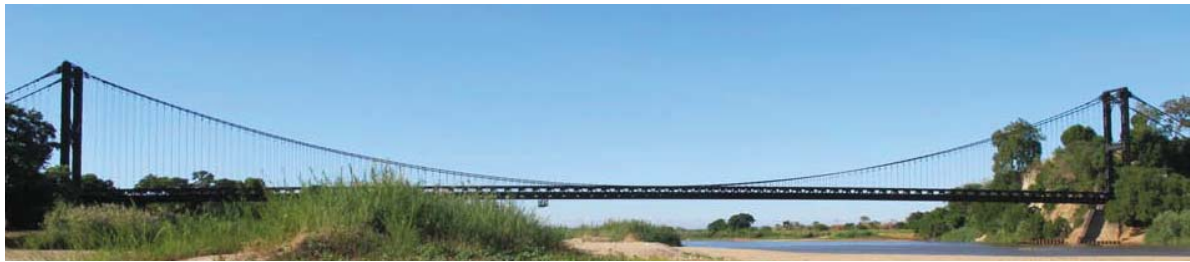
Figure 1. The Kamoro Suspension Bridge
