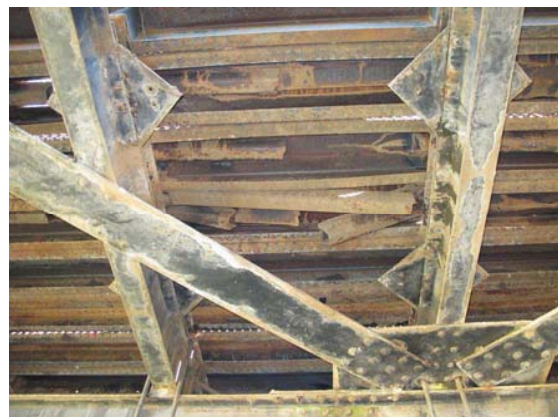
Figure 5. The underneath of the orthotropic deck.
