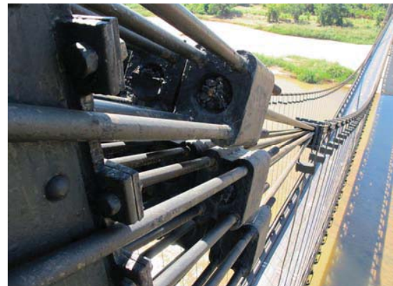
Figure 3. Cable anchorages on towers.
