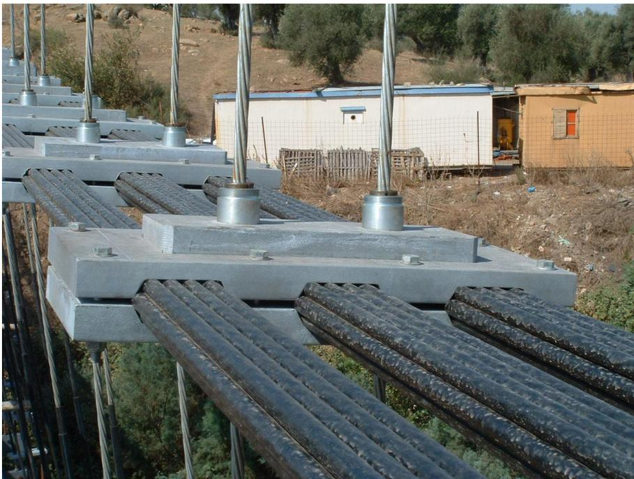
following a philosophy developed for larger bridges by William Brown (1928-2005) were the saddles are an assemblage of smaller components made of rolled and welded plates instead of being made of a single casting. The old saddles have been encased in a steel box, cement grouted once the old cables and stays were removed. The new saddles are placed on top of these encasings on Steel-Teflon bearing pads that allow longitudinal displacements.
