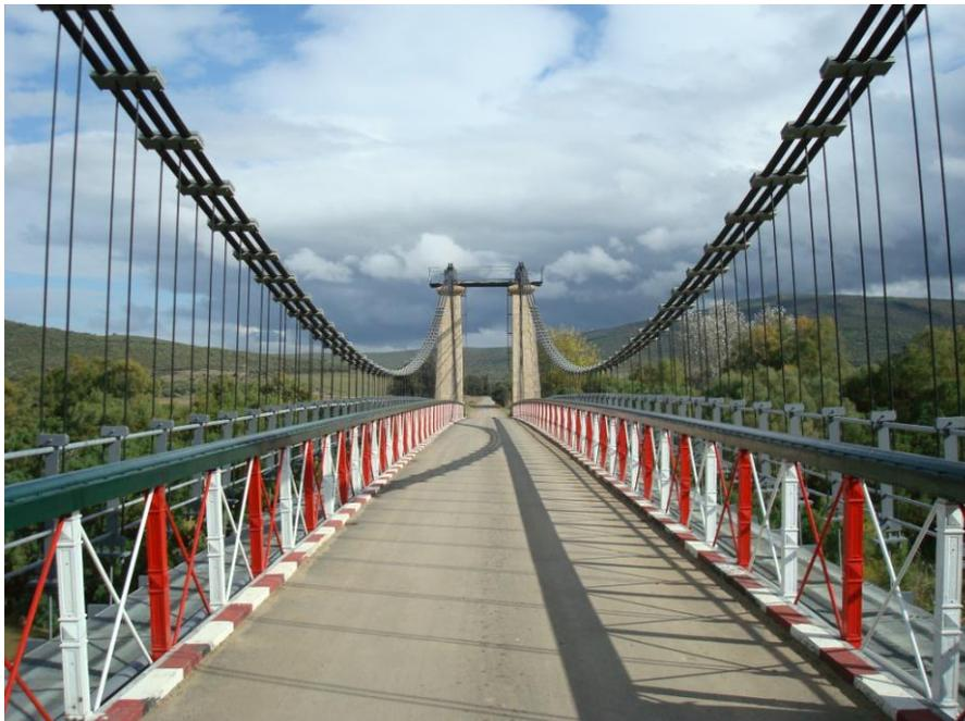
accounted for when designing the new suspension system thus obtaining a stiffer structure (via the increased tension in the cables) but also a tougher and more ductile response of the deck under the increased live loading of today traffic.
