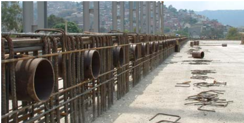
Photo 6: The launching concrete girders steel reinforcements
