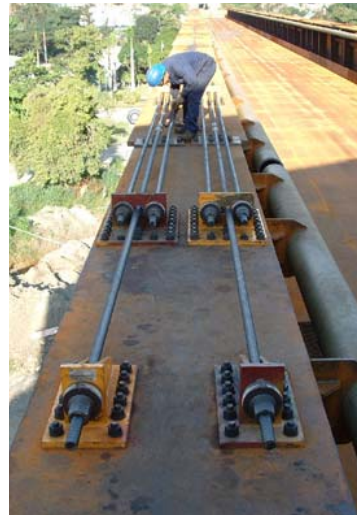
Photo 3: Top Flange connection
