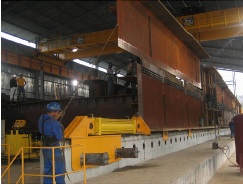
Photo 5: The launching yard
