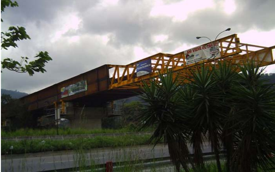
Photo 7: The launching phase over the motorway
