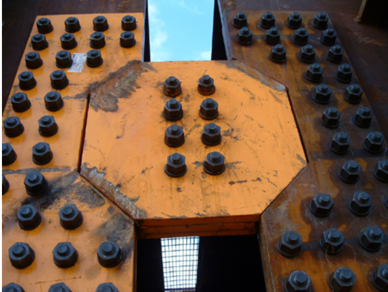
Photo 2: Shear key
