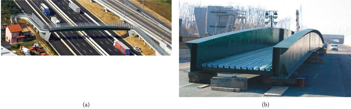
FIGURE 1: Pregnana footbridge: (a) in-service overpass on the TO-MI highway; (b) preassembly of steel beams and deck for the main span.
