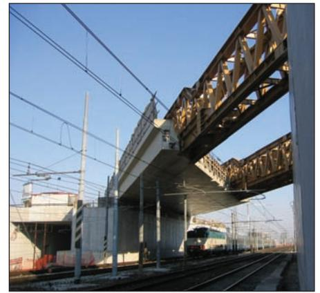
Fig. 4: The first slab halfway through launching, rail traffic unaffected
