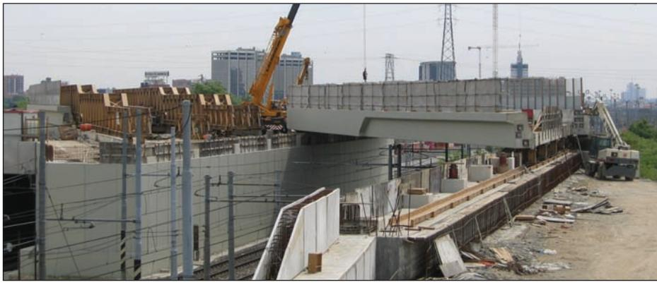
Fig. 6: The first slab is skidded along the abutment into its final position
