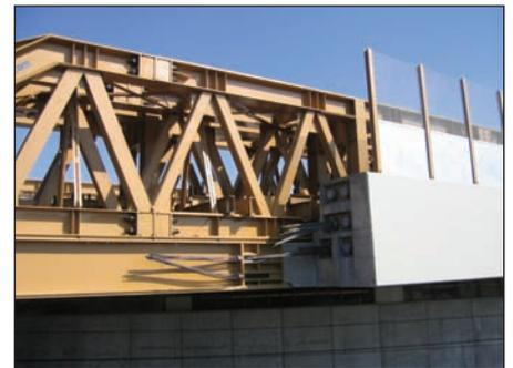
Fig. 5: Front connection between the launching girders and the slab
