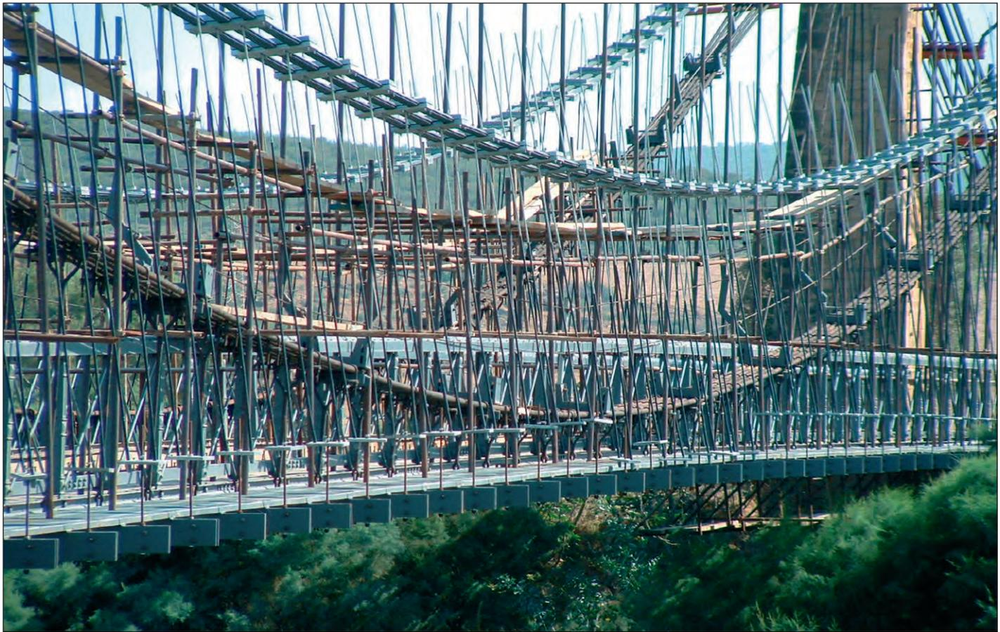
Fig. 12: The two suspension systems before the load transfer
