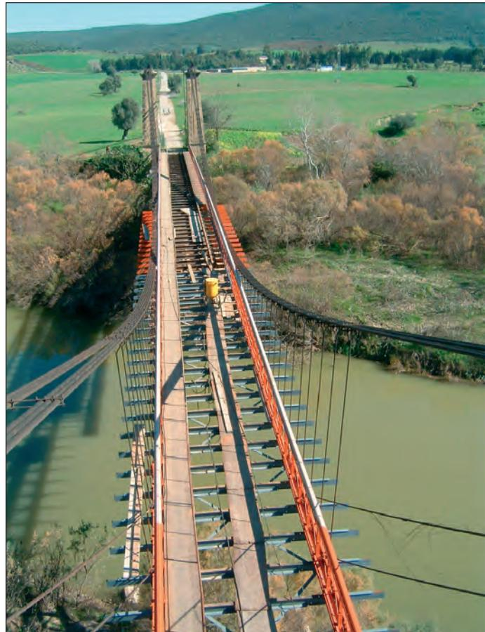
Fig. 11: Strengthening and widening the transverse beams
