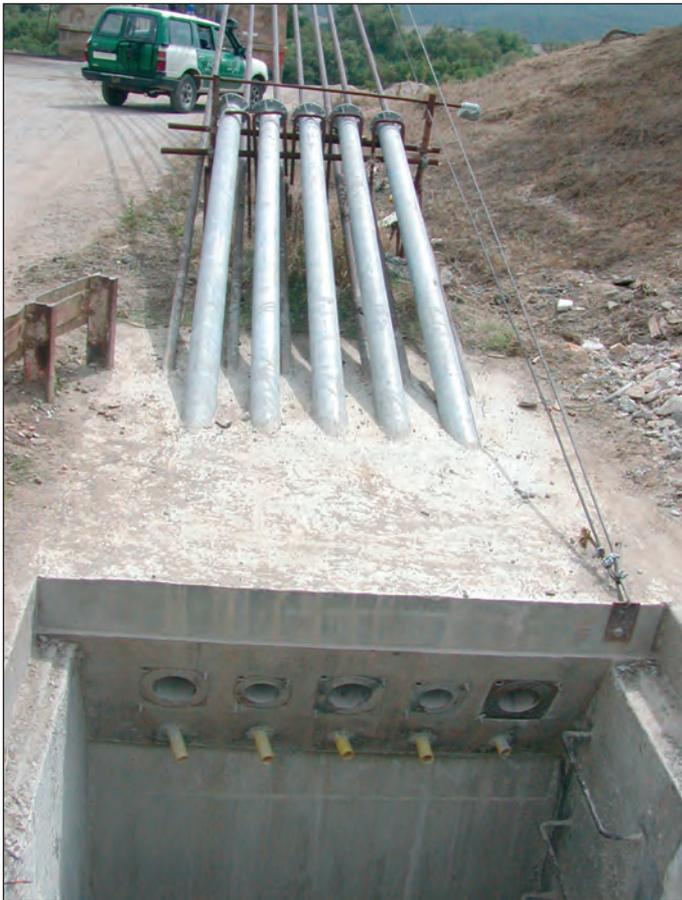
Fig. 10: The new anchorages cast inside the existing ones
