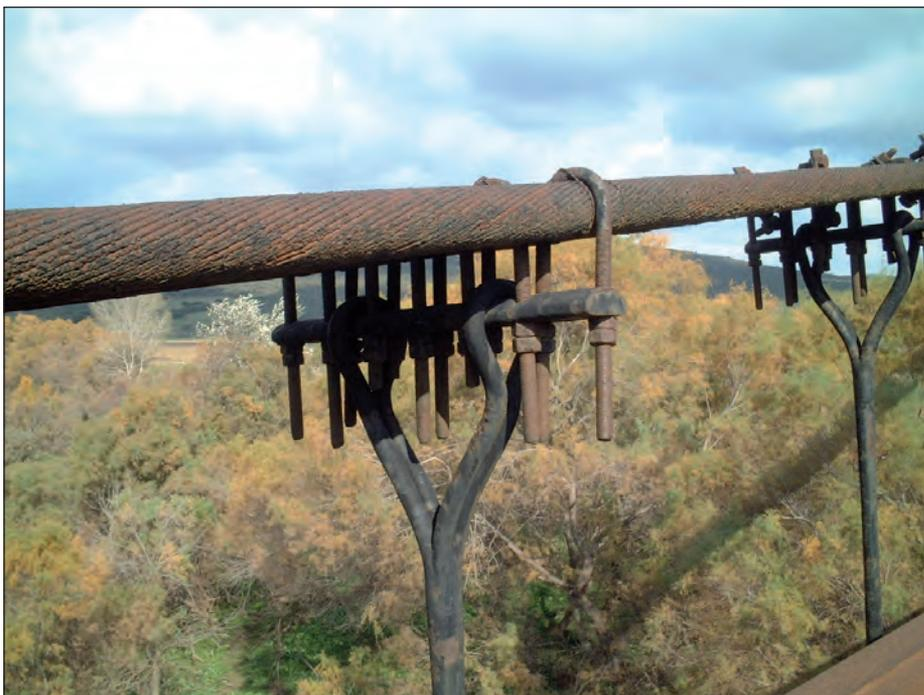
Fig. 3: Cables, clamps and hangers
